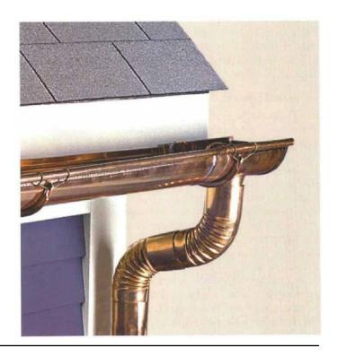
rigidly anchored on both ends, such as one that rounds two corners, is subject to expansion and contraction woes. Temperature-induced expansion or contraction can cause the gutter to wrinkle, or stress the seams, possibly to the point where the seal breaks and leaks begin.
